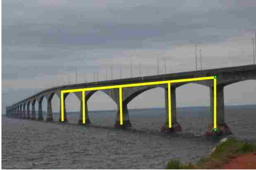
Figure 2.4a Application of Column-Beam Frame on a Bridge
